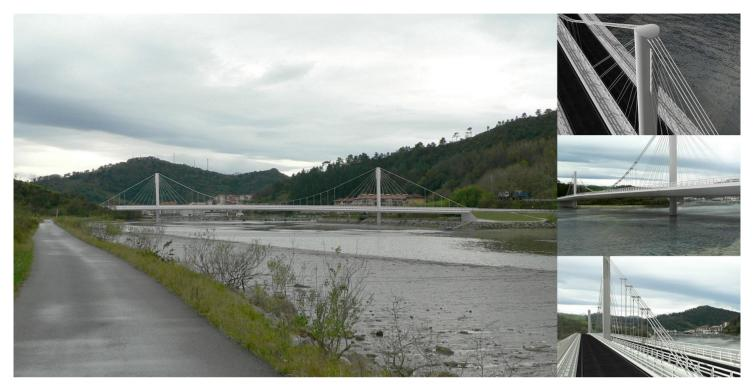
The bridge which crosses the Orio River employs a hybrid support system combining suspension with cable-stayed. The aim of such a system is to decrease the height of the piers and to create a structure which is less aggressive with the surrounding scenery and at the same time, lowering the costs of a traditional suspension bridge construction. The bridge has a main 170.0m span with 60.0m compensation spans which more than cover the boat race channel.
